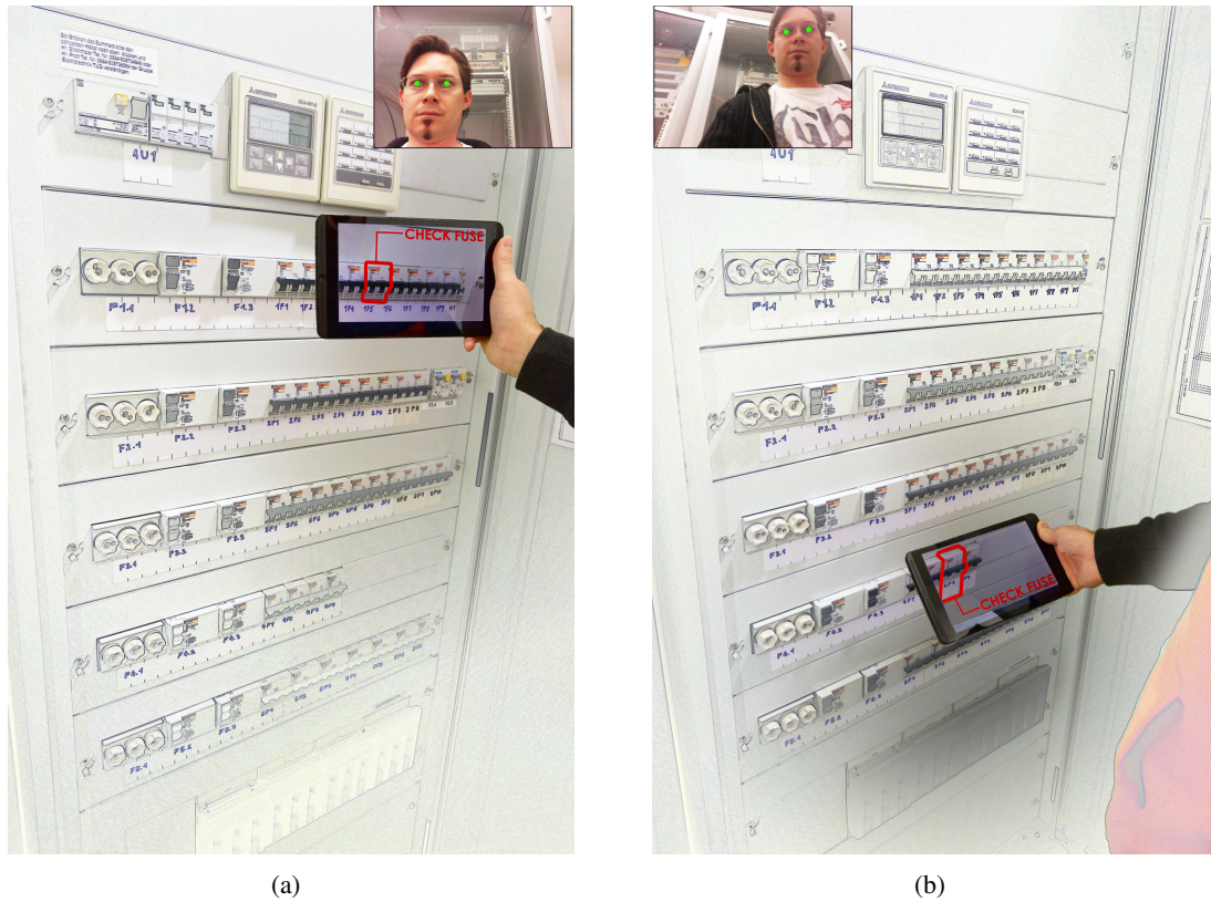
Figure 1.7: Augmented Reality Documentation on a Handheld Device. In a typical usage scenario, the user moves the handheld device from one position (a) to another (b) to view different AR instructions. The resulting transition of the user’s head pose, in relation to the device, requires updating the viewing frustum.
